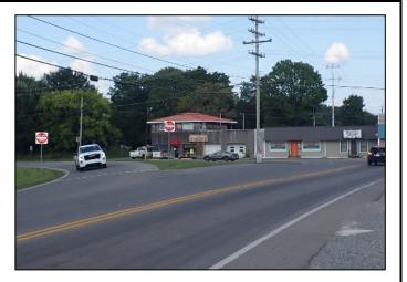
Improvement Concept: An improvement option is to remove the channelized right-turn and square up the intersection. Future phases of the project would determine if a right-turn lane is necessary and if the intersection could be converted to a three-way stop-controlled intersection. A turning movement count would be needed to analyze the traffic impacts.
